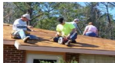
Bob Installing new roof with fellow crew members
